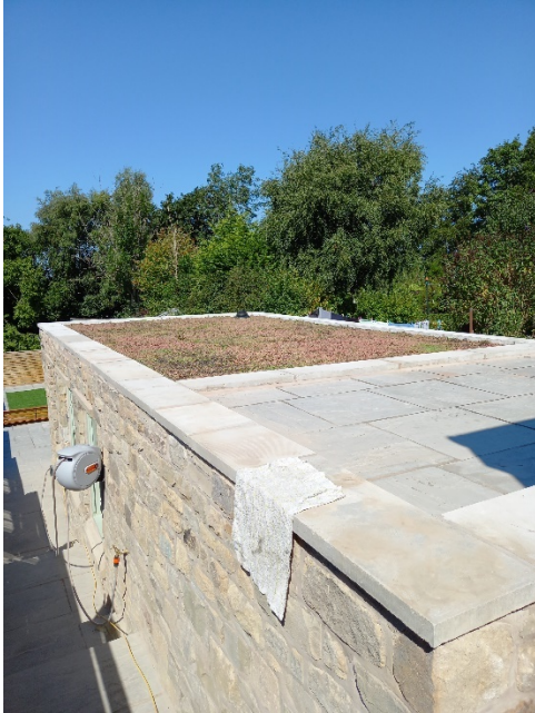
View of roof from east
